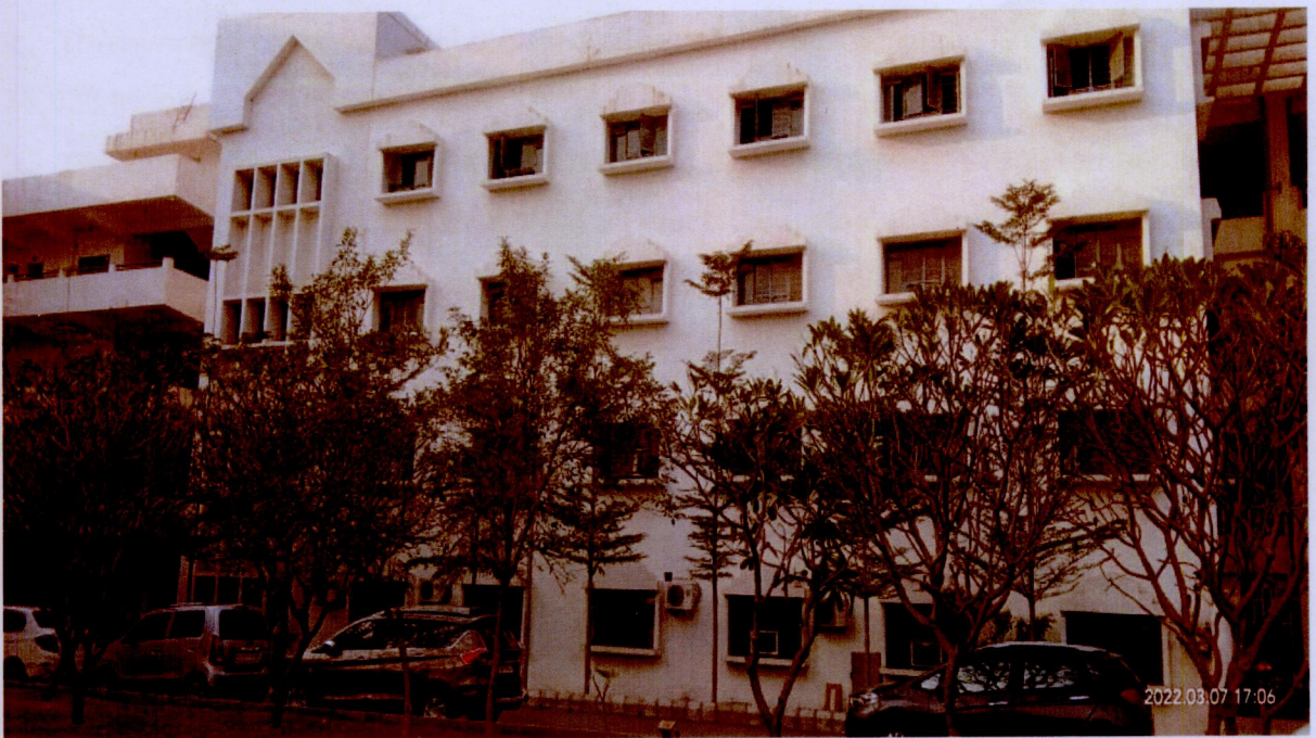
Annex Building B
